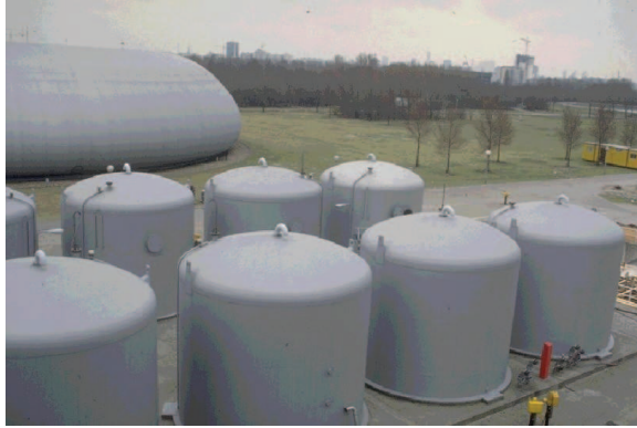
Figure 26 - Cylindrical steel pressure filters
