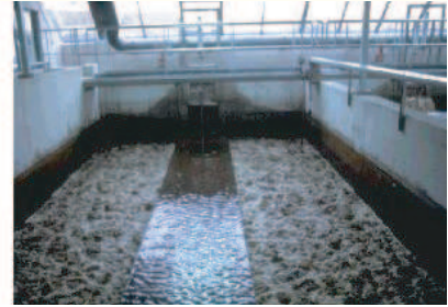
backwashing with water and air
