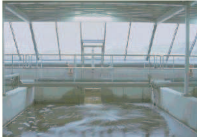
Figure 8 - Filtration, backwashing with water and air
