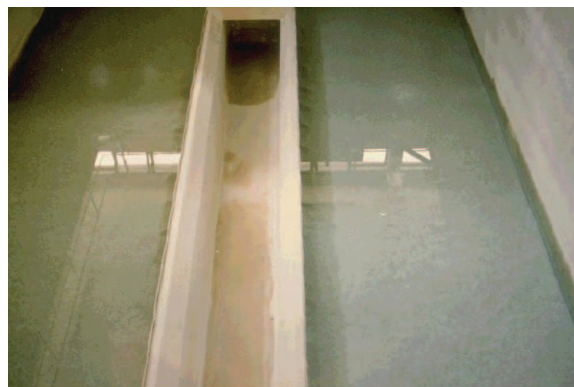
Figure 14 - A central backwash trough
